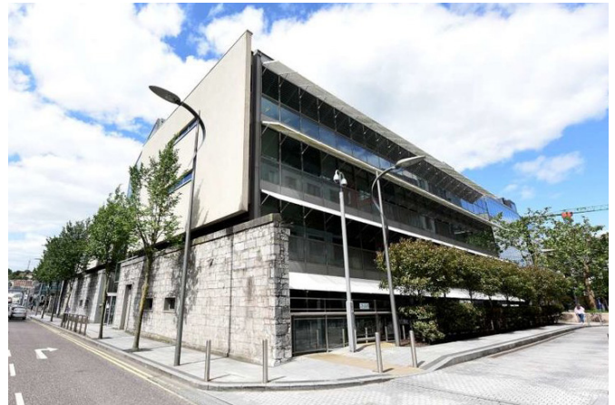
Office property in Cork, Ireland
