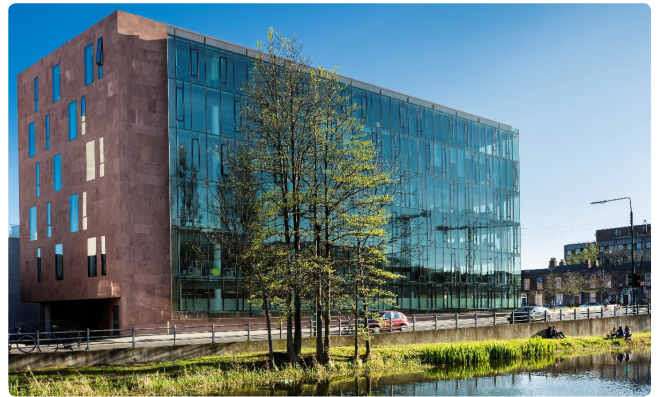
Office property, Dublin
